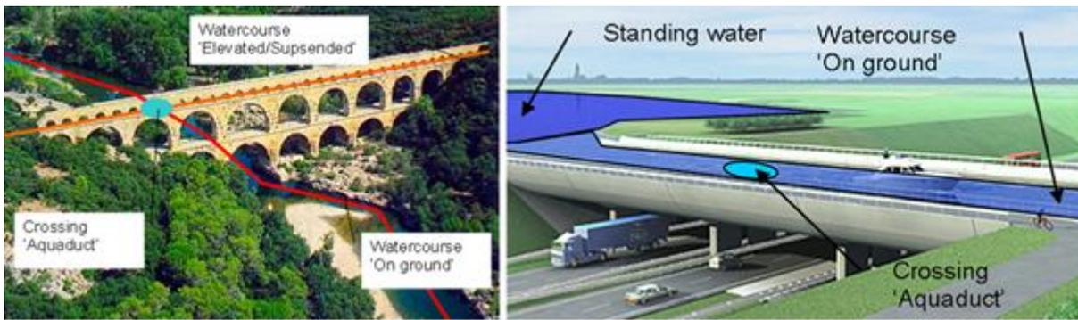
**Figure 37 – Aquaduct with two watercourses crossing each other (source: [www.leestrainer.nl](http://www.leestrainer.nl)) and aquaduct crossing a road (water still on ground level)**
