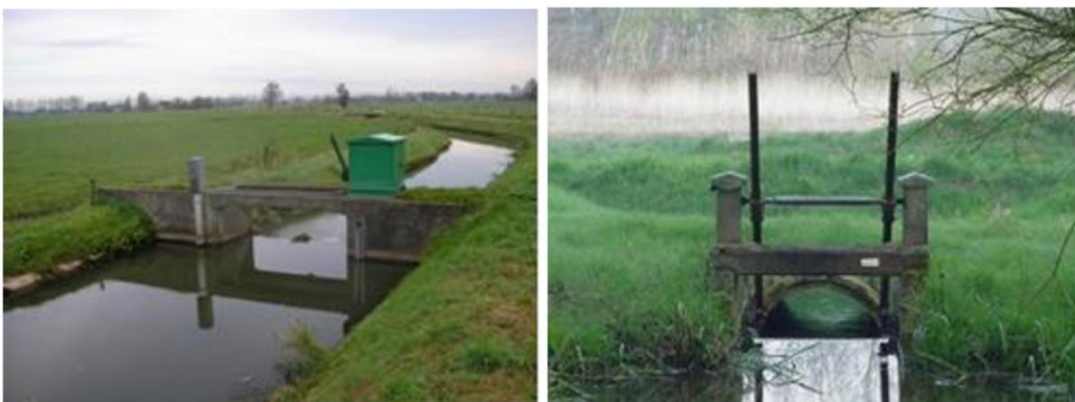
Figure 20 - Small weir (left) and sluice (right)
